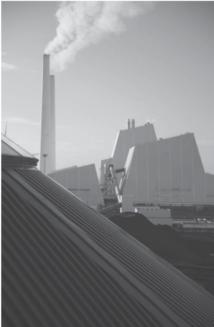
FIGURE 1.1 The Avedøre Power Station, Denmark.
